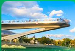
Floating Bridge Moscow
